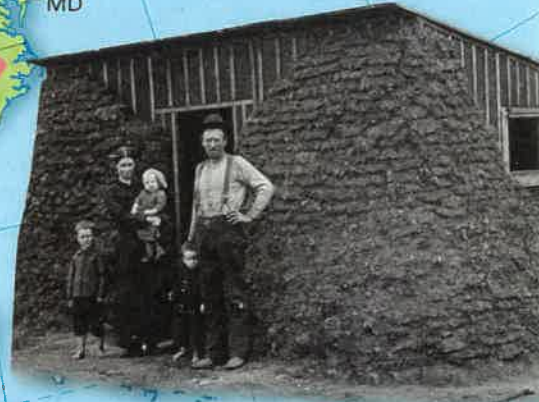
▲ A family stands outside their sod house on the Great Plains in 1880. There were very few trees on the Great Plains, and wood was expensive because it had to be shipped to the region. So settlers cut chunks of earth from the ground to build their homes.
