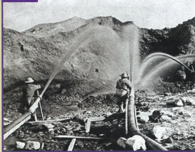
▲ The high-pressure water washed the loose earth into large sluices, or ditches that carried the water and earth into riffle boxes. The boxes agitated the water, causing the silver or gold to settle out. The leftover debris, called tailings or “slickens,” was then washed into a nearby stream.
