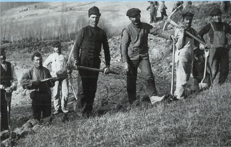
▲ Many Italian immigrants took jobs as construction workers, bricklayers, and dockworkers in urban areas, but this group is building a railroad, c. 1900.
