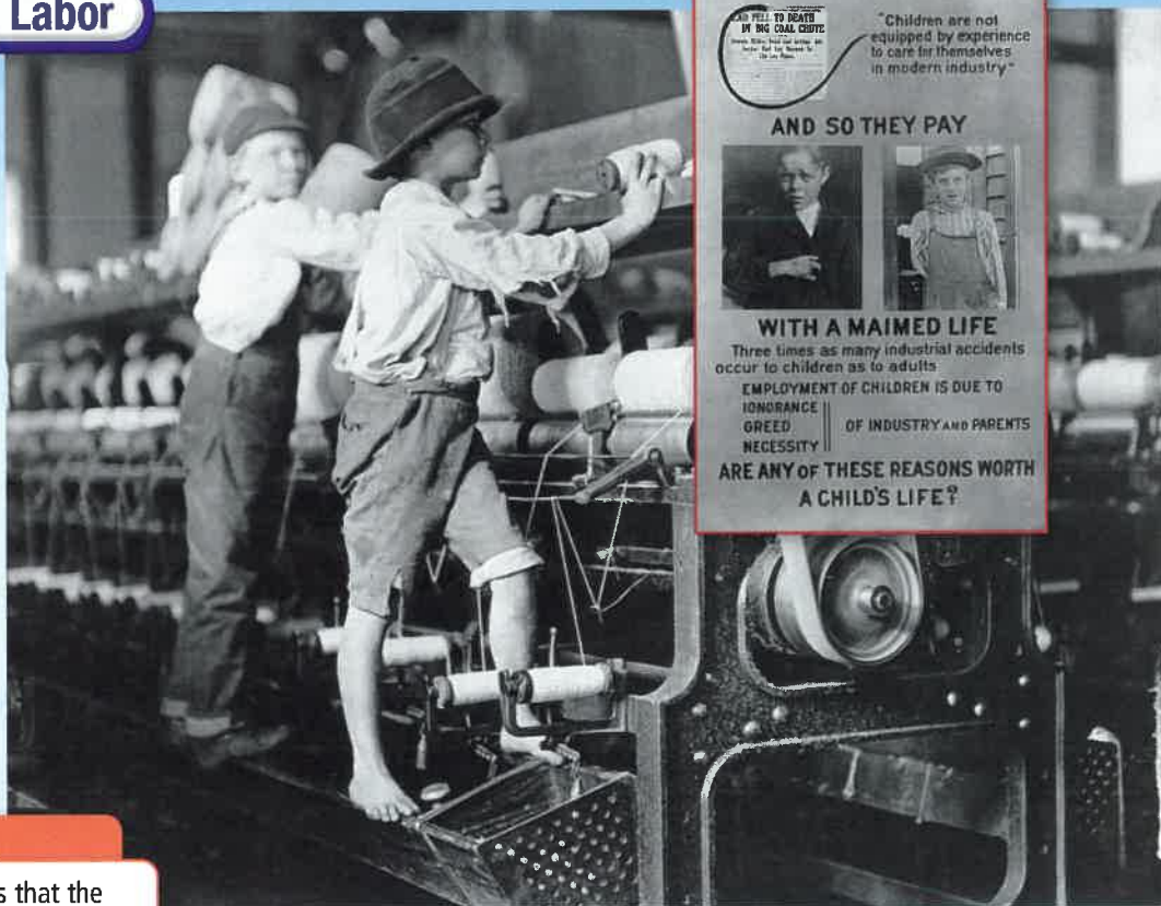
▲ At a Georgia cotton mill in 1909, two boys keep a spinning machine running by repairing broken thread and replacing bobbins as they are filled.
